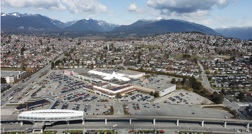
Aerial view of Brentwood Town Centre prior to redevelopment with the SkyTrain station in the foreground. Photo Credit: Shape Properties Corporation
