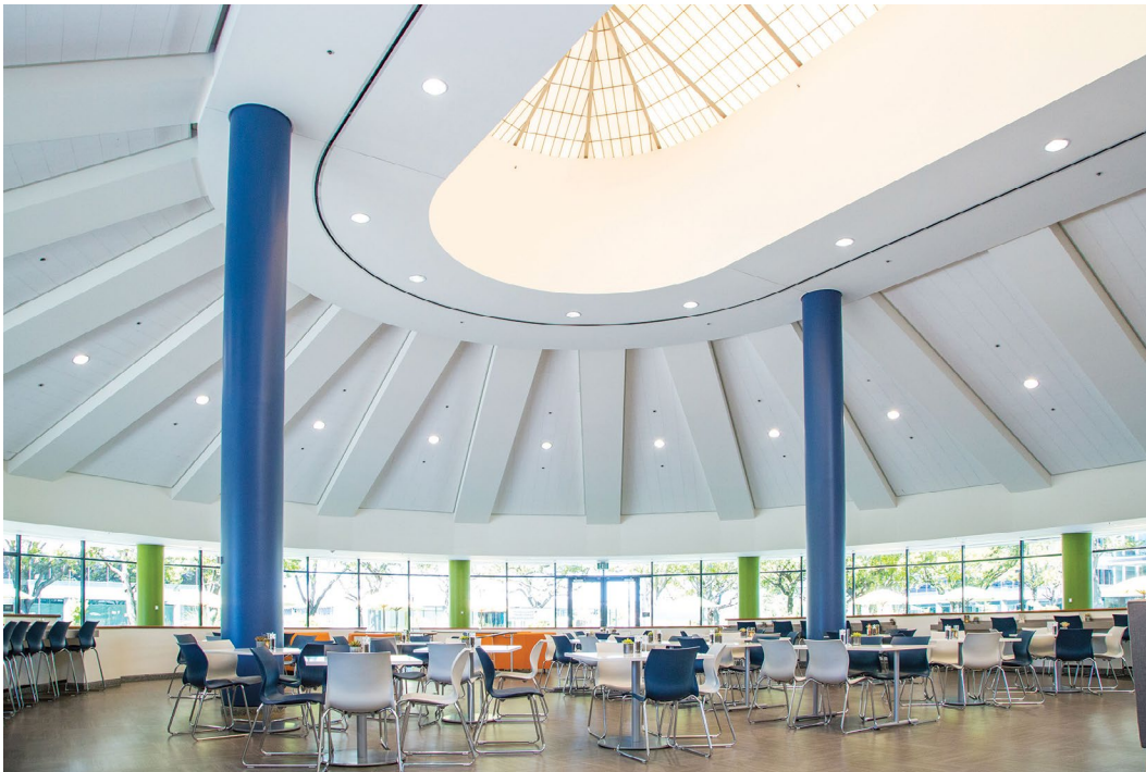
A conference center and cafeteria dating back to Rosewood Commons' days as a single-tenant corporate campus were remodeled to provide those working on-site with additional places to meet.
