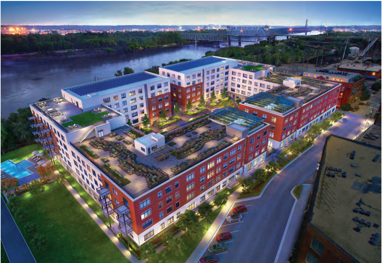
At 276 units, Second + Delaware, in Kansas City, Missouri, claimed to be the largest passive-building multifamily project in the world when it opened in 2020.
