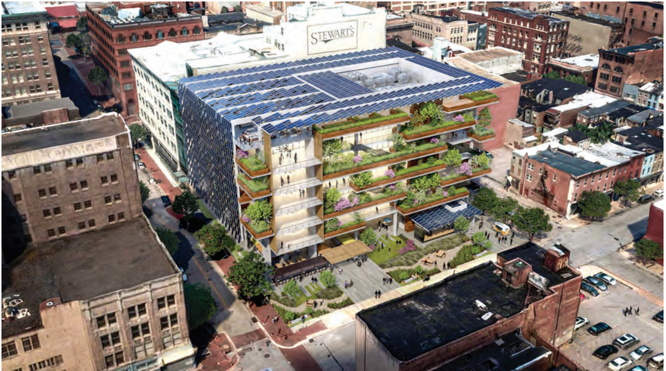
Gensler's morphable office concept for a hypothetical site in Baltimore. It features movable walls that can open on two sides to allow fresh air in, as well as an exterior walking path on each upper floor.
