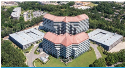
Southern Company Energy Center BIRMINGHAM, AL
