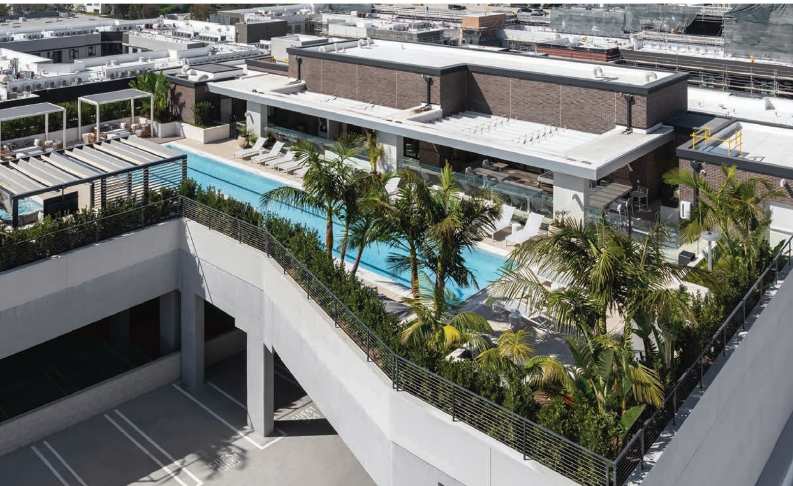
Rooftop decks with pools and lounges were added to the garages at the Row at Red Hill, helping to create a leasing differentiator.
