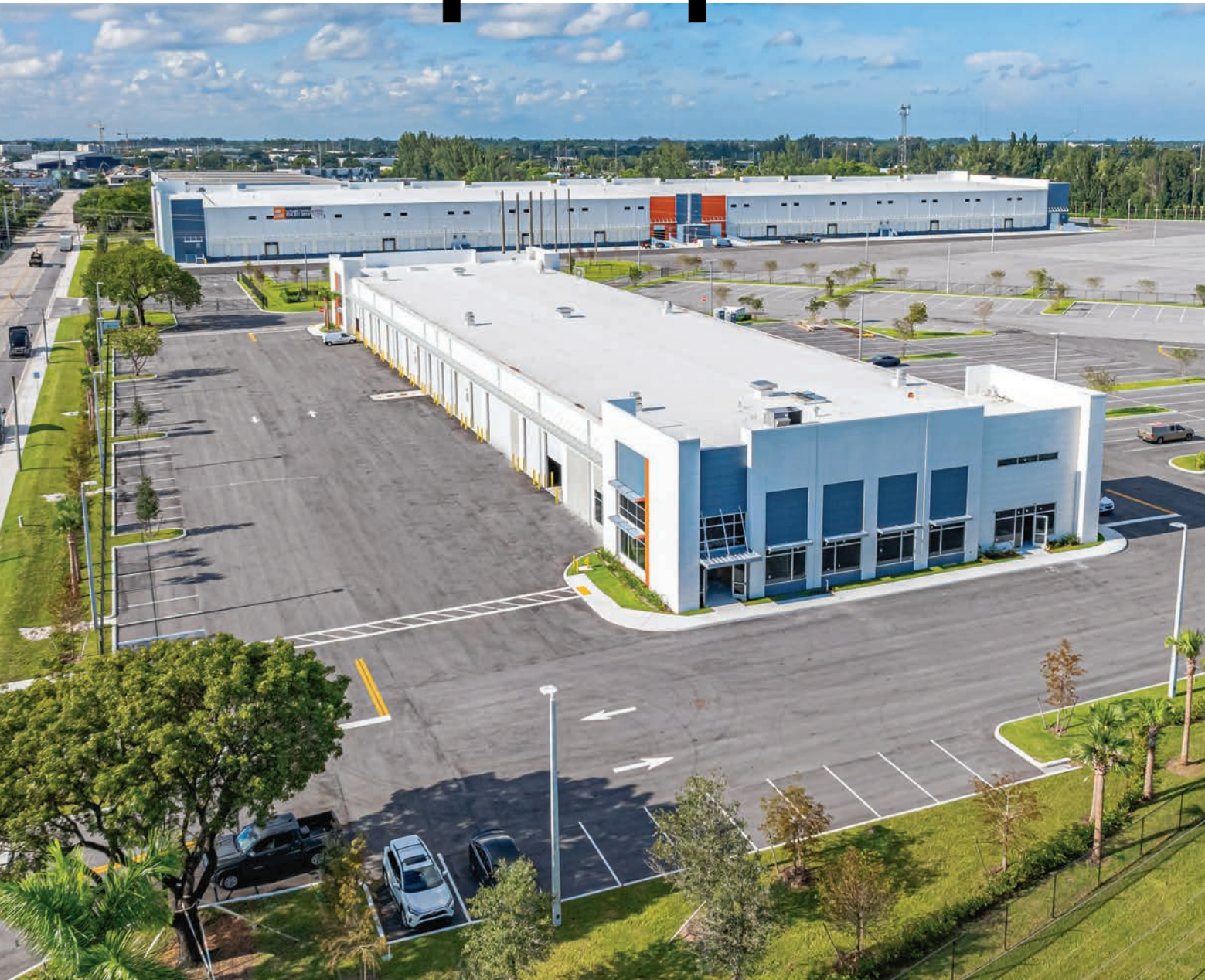
Industrial Outdoor Ventures' Davie Industrial Center in Davie, Florida, includes a 183,833-square-foot spec distribution building with 11.5 acres of outdoor storage available for lease. An adjacent 42,866-square-foot service building is leased to Doka USA.
