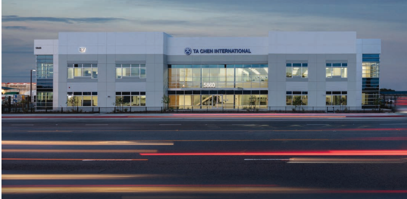
CenterPoint Properties delivered a build-to-suit distribution facility near the Port of Long Beach in California that also serves as the U.S. headquarters for Ta Chen International Inc. The 129,300-square-foot Class A facility includes a two-story, 42,700-square-foot office, four docks, three drive-ins, a 32-foot clear height and parking for 164 cars.
