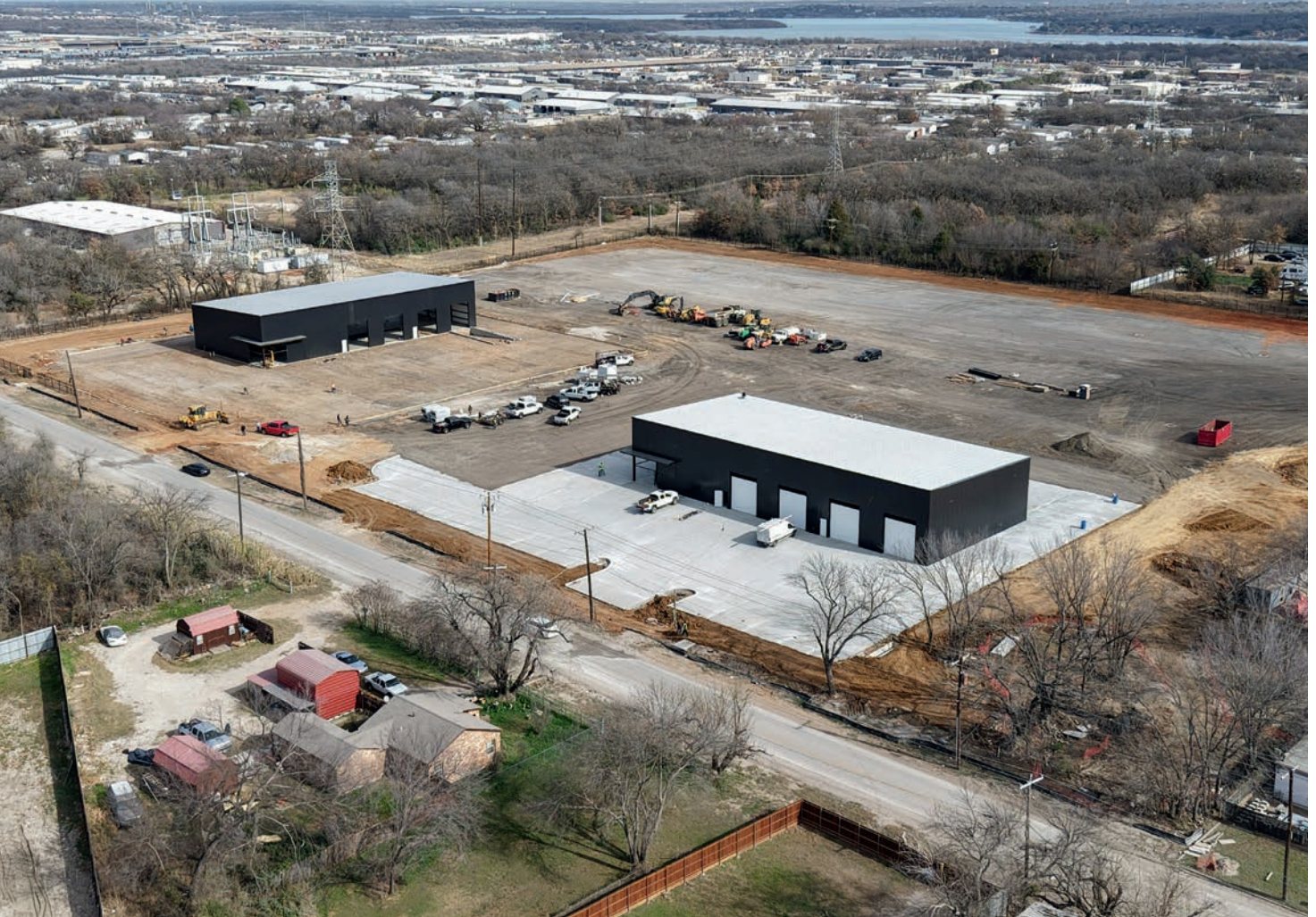
CanTex Capital's speculative IOS development at 4729 Mansfield Highway in South Fort Worth, Texas, features two 5-acre sites, each with a 10,500-square-foot building.
