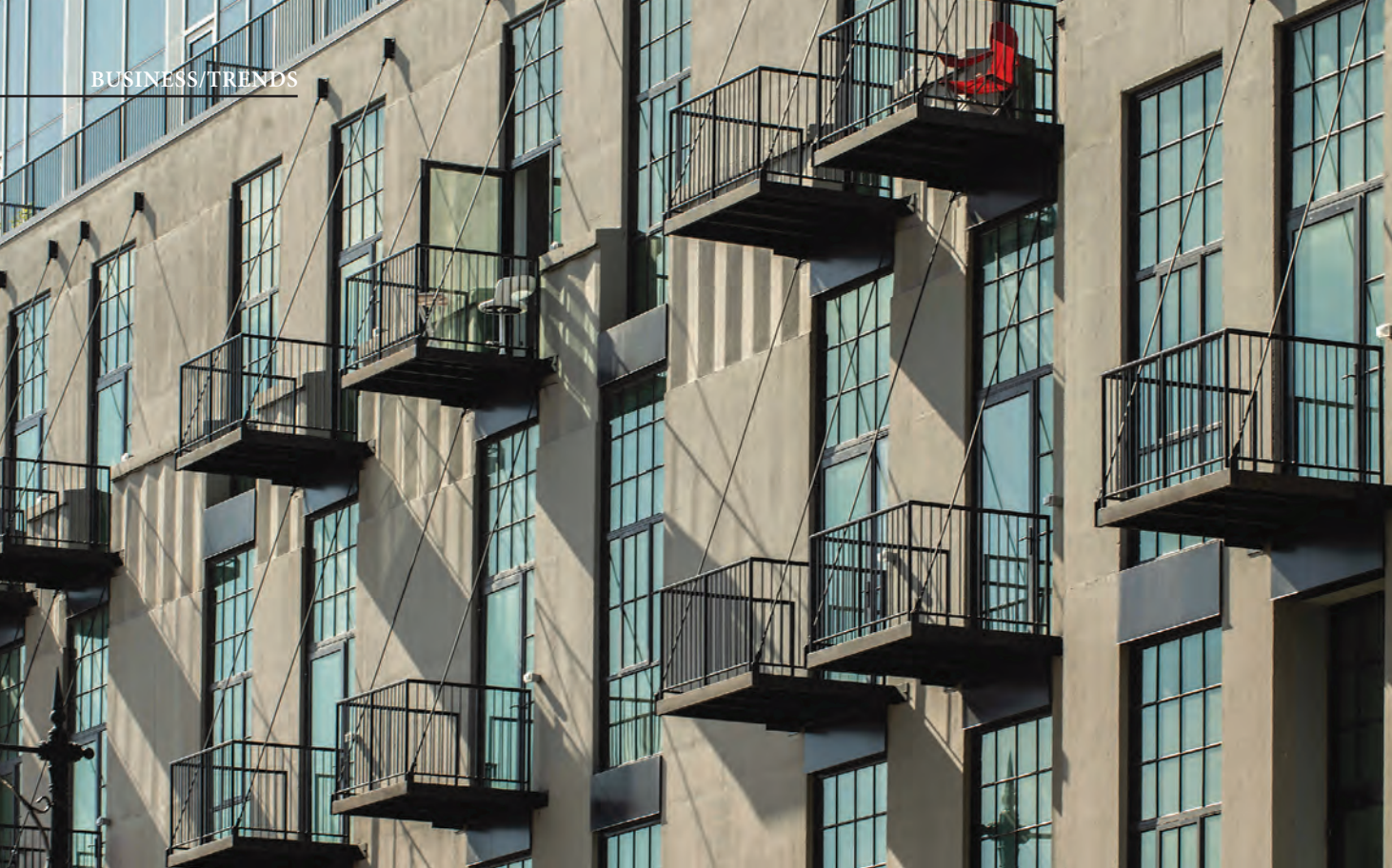
Decorative elements found in the original building were turned into balconies at 6 Corners Lofts to provide each residential unit outdoor space.
