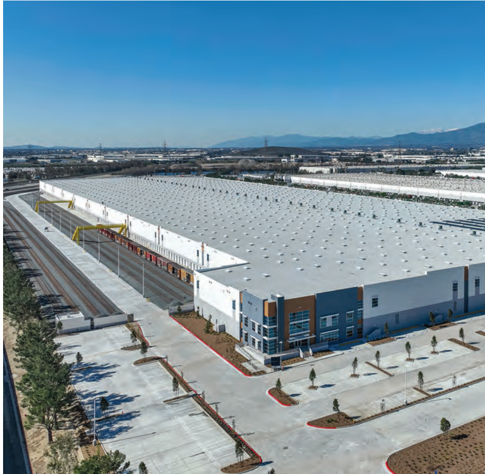
The Palmer's Oak Logistics Center project involved the redevelopment of a former U.S. Army supply depot and construction of nearly 3 miles of rail across eight spurs.
