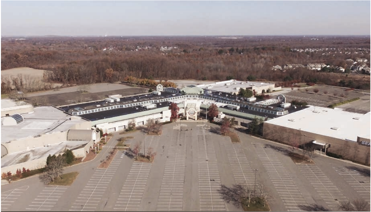
Clarion Partners and MRP Industrial acquired the Burlington Center mall site for redevelopment in 2019.
