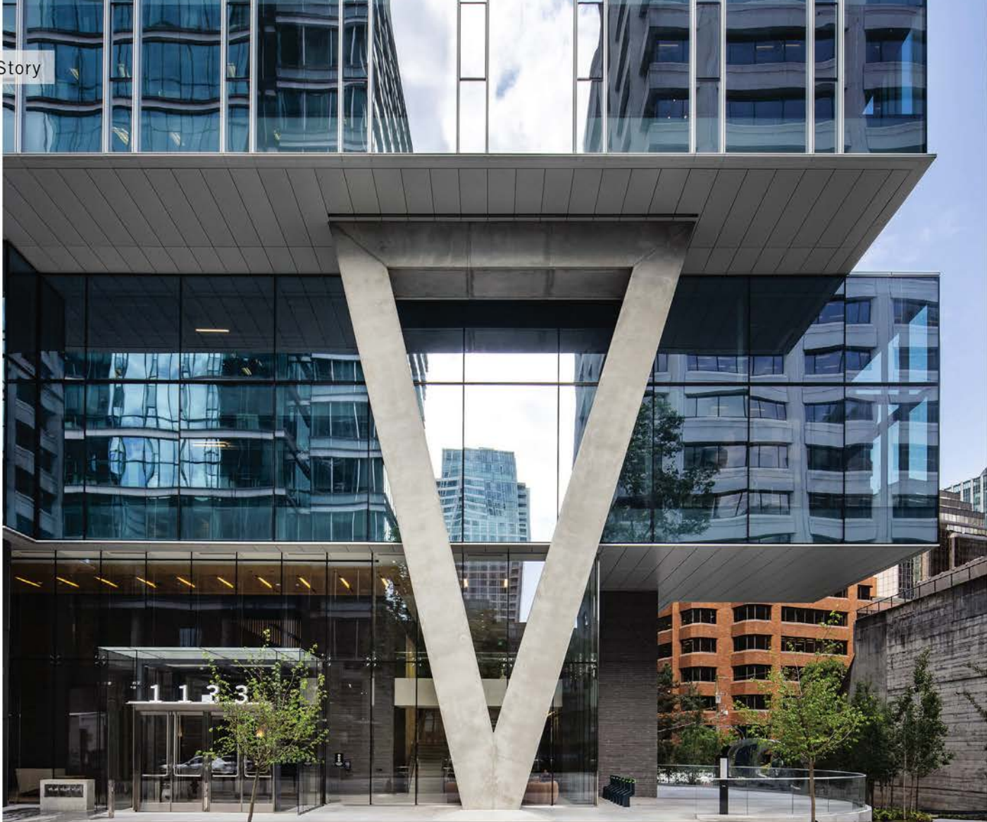
The Stack's zero-carbon framework includes low-carbon building systems, a triple-pane curtain wall and an enhanced rainwater management system.
