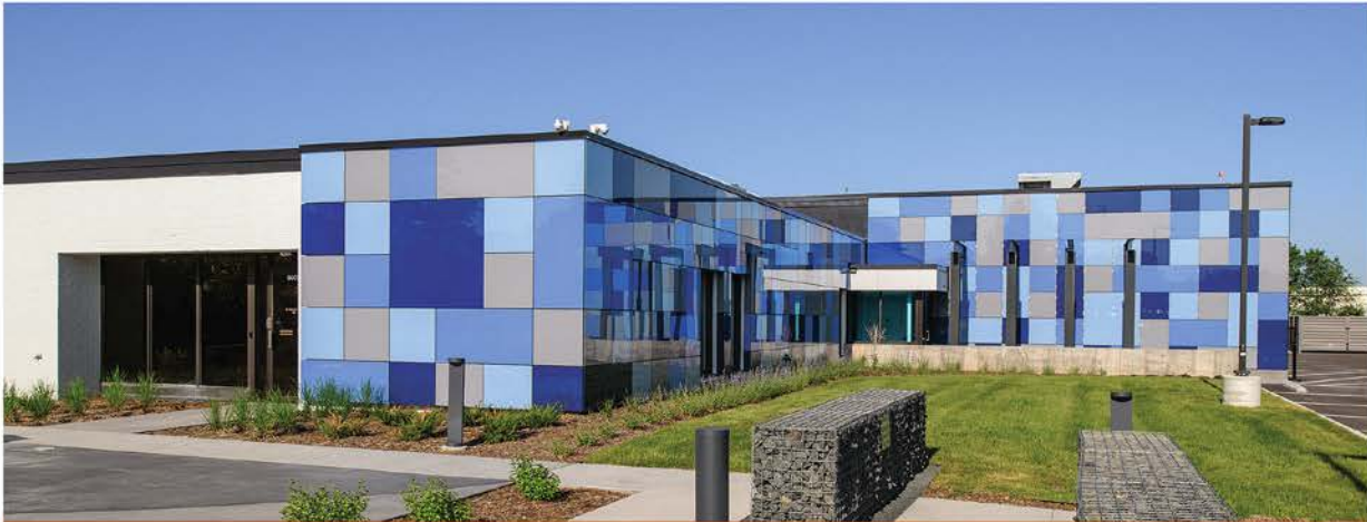
The cladding solution for the Cafesjian Art Trust museum was chosen both for its performance and its aesthetics.
