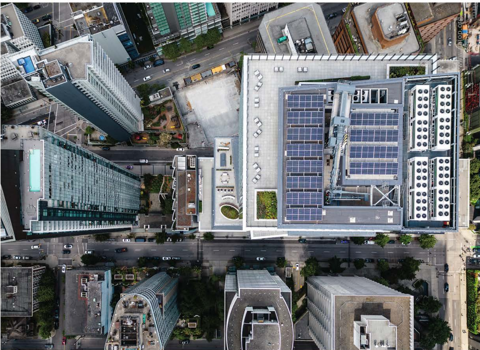
An overhead view of The Stack shows the office tower's rooftop photovoltaic solar array.
