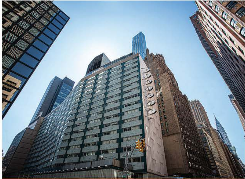
An 800-key Hilton Doubletree was converted into an apartment complex in Midtown Manhattan for students at LIM College.
