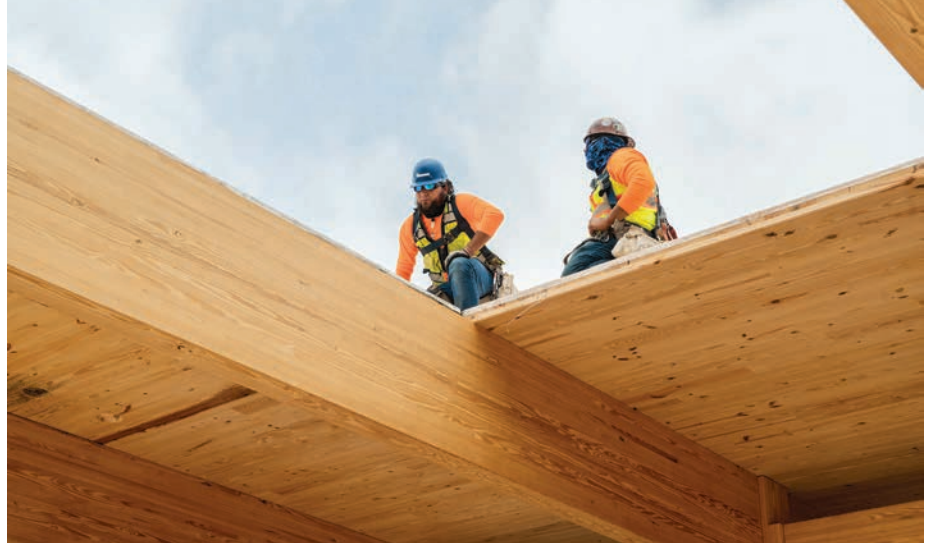
Assembling 619 Ponce’s mass timber superstructure.
