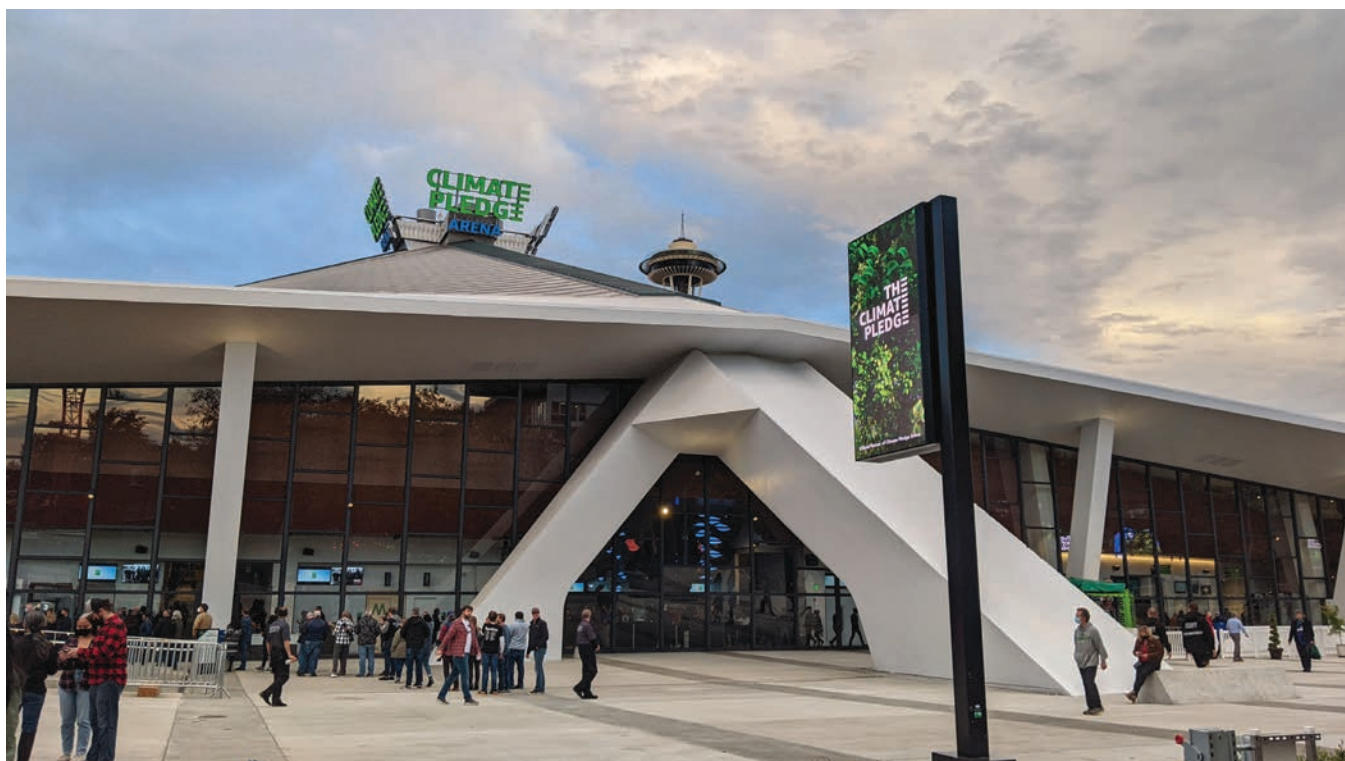
An exterior view of one of the buttresses supporting the landmark roof at Climate Pledge Arena.
