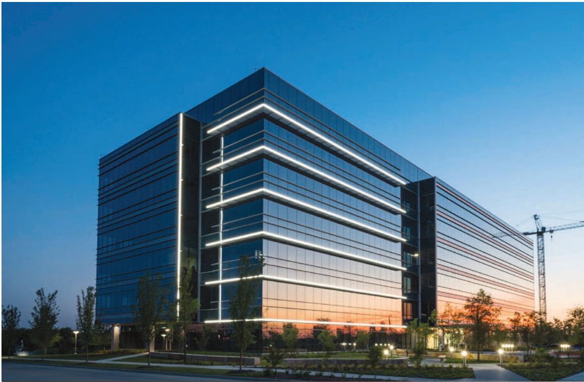
The Offices Two at Frisco Station in Frisco, Texas. VanTrust has invested more than $250 million in this award-winning 242-acre mixed-use development north of Dallas.
