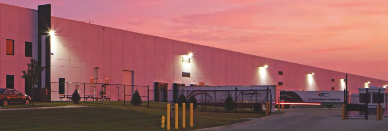
The 996,930-square-foot Cooper Tire and Rubber Co. warehouse and distribution center in Whiteland, Indiana. Mohr Capital broke ground on the project in June 2020, and it was ready for occupancy in January 2021.
