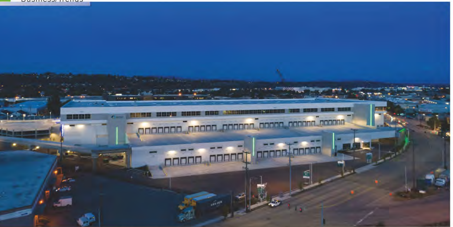
Seattle's Georgetown Crossroads at night. The Prologis-designed 590,000-square-foot, 14-acre development has more than 100 docks and 635 parking spaces.
