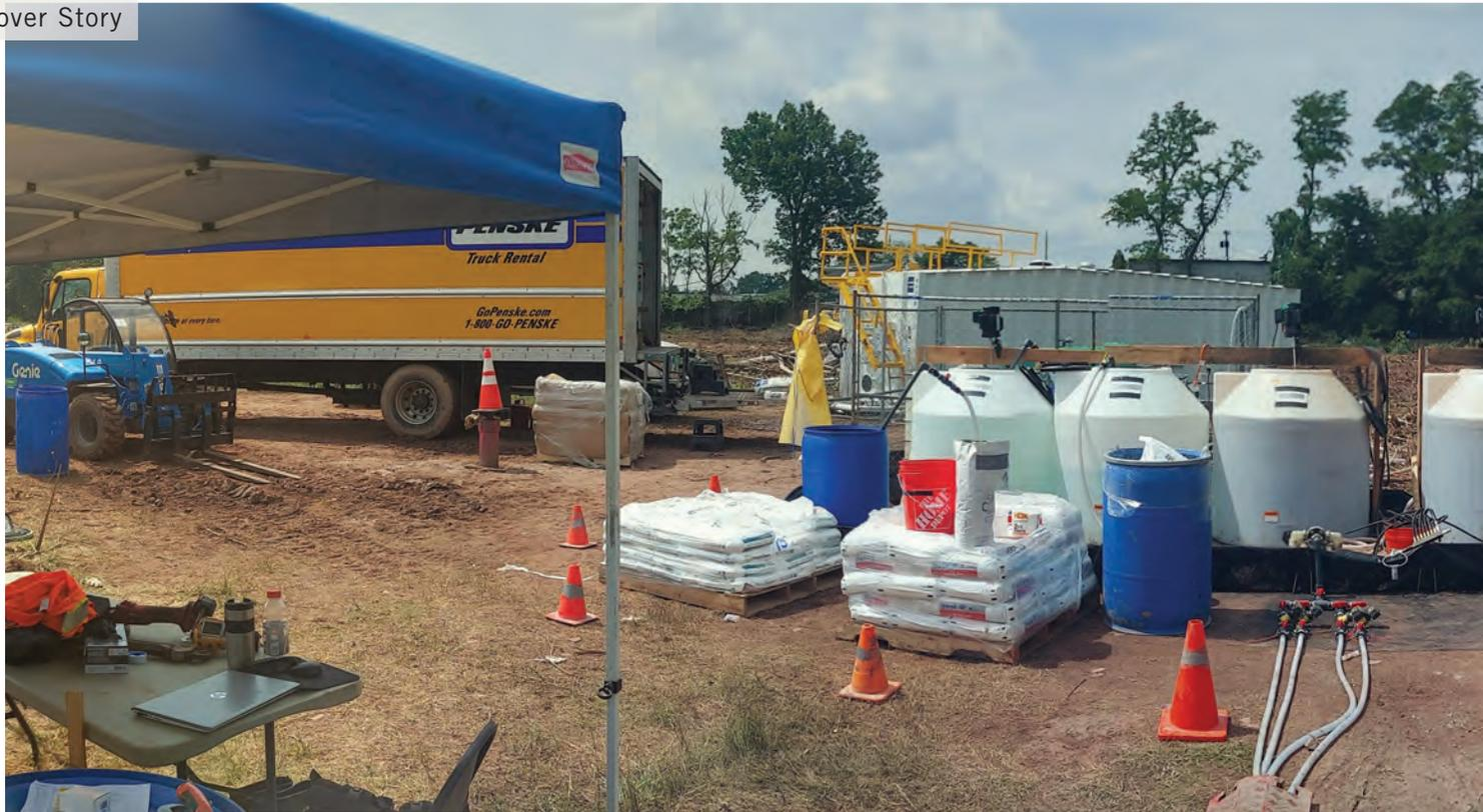
Injection pumps and mixing tanks are used to conduct in-situ chemical oxidation of contaminants at Bridge Industrial's project in Belleville, New Jersey. The site is within six miles of the Lincoln Tunnel, a major artery into New York City.
