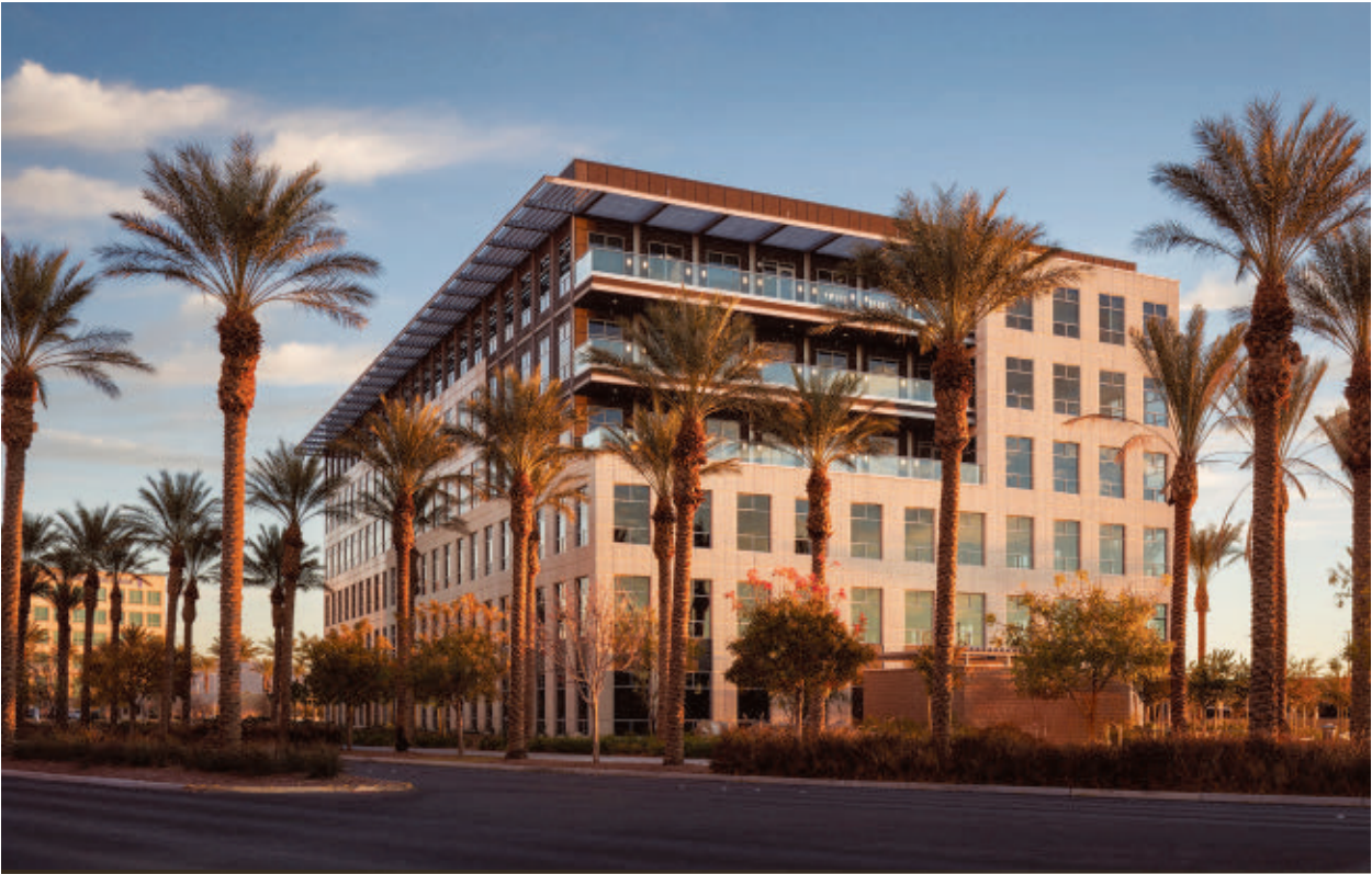
The executive office balconies at Two Summerlin, located on the fourth through sixth floors, offer views of the Las Vegas Strip and the Red Rock Canyon mountains.
