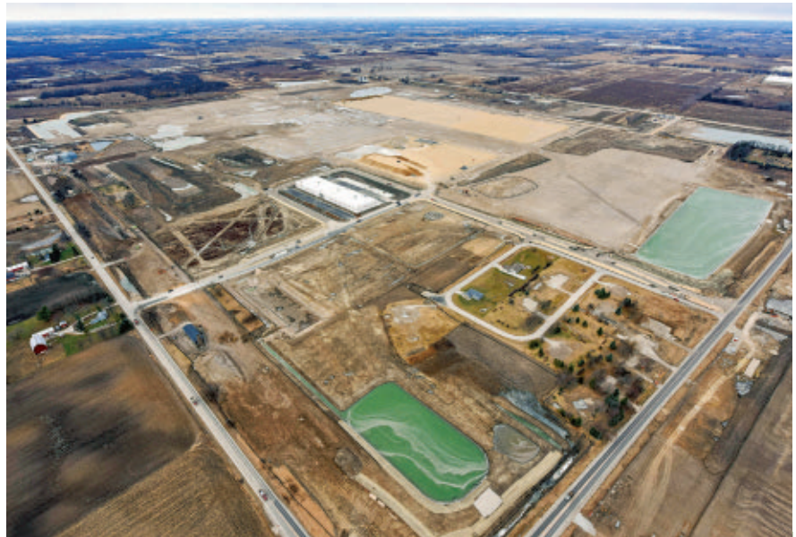
As this aerial photo from January shows, development is well underway at the Foxconn site in southeastern Wisconsin. It's one of the largest corporate attraction projects in U.S. history.
