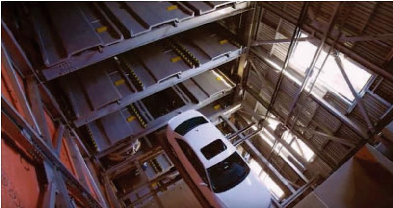
The seven-story Hive Parking Structure, the first and only fully automated parking system in the San Francisco Bay Area, accommodates 39 cars on a 1,600-square-foot site, room for only seven standard parking spaces.
