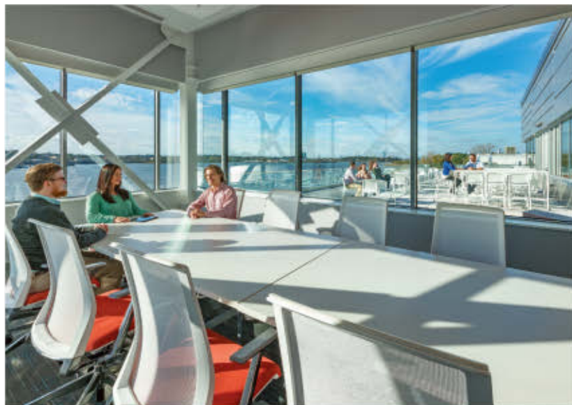
The design transformed an outdated warehouse building into an attractive, energy-efficient and natural light-filled office and fulfillment facility; the project was a major part of the Boston Scientific Global Facilities Master Plan.
