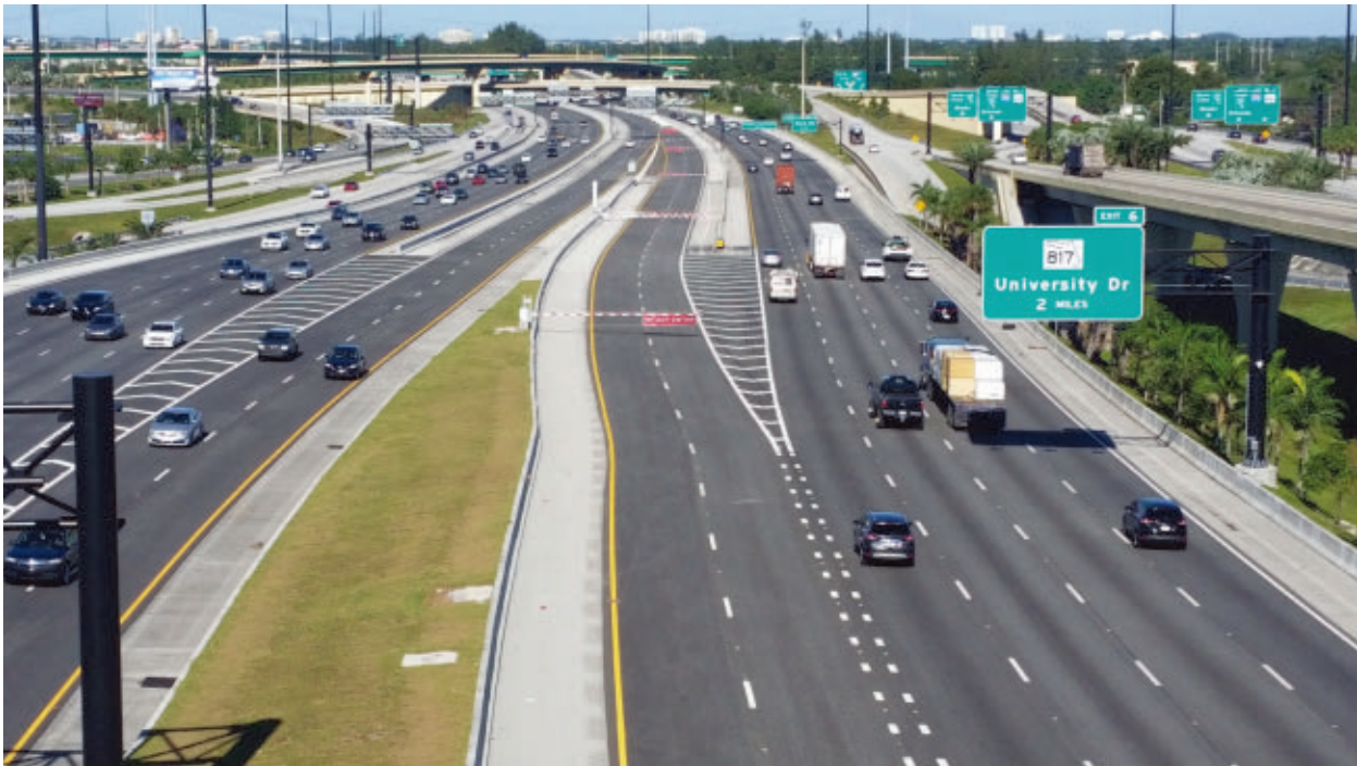
The reversible toll lanes known as 595 Express have eased traffic congestion between Ft. Lauderdale and its western suburbs in South Florida. The lanes were constructed by a P3 between the Florida Department of Transportation and ACS Infrastructure Development Inc.
