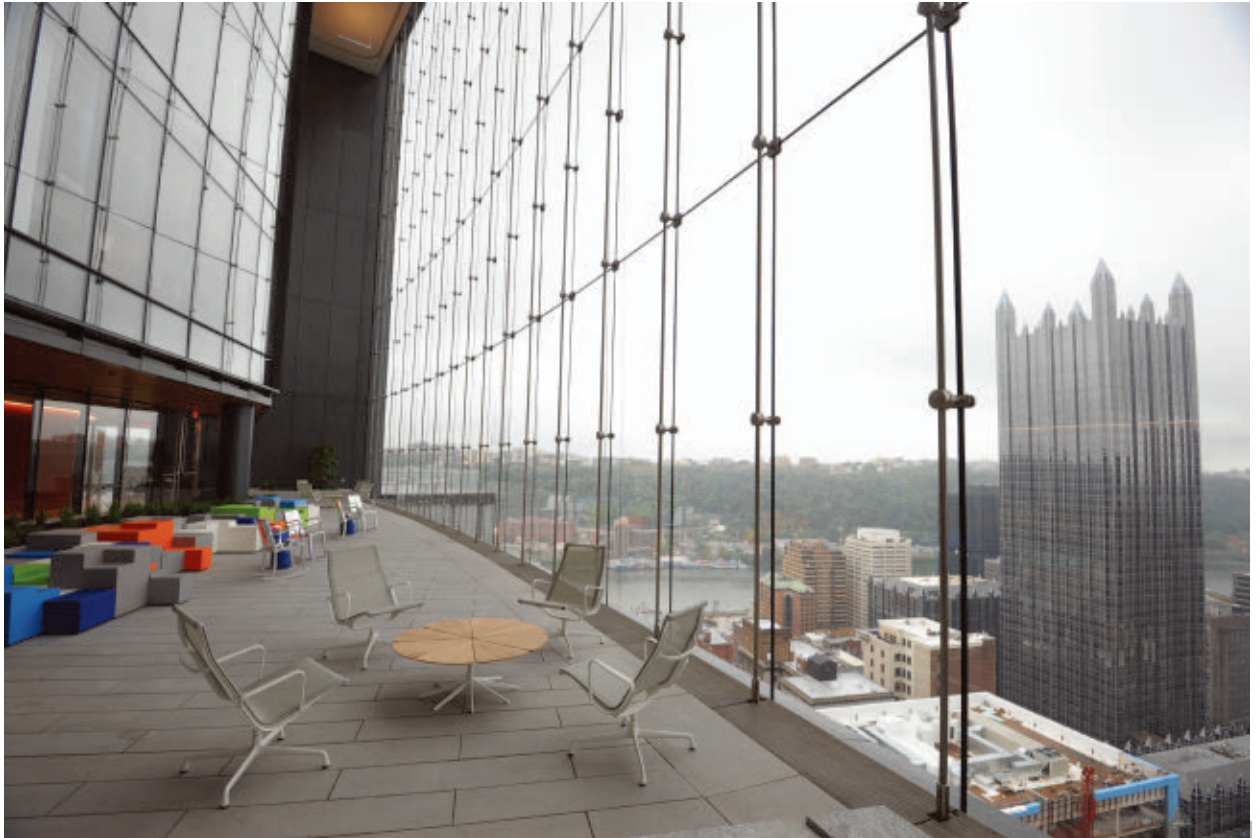
The Tower at PNC Plaza, PNC Financial Services Group's world headquarters in Pittsburgh, features a passive ventilation system that brings fresh air into the building via a solar chimney and a double-curtainwall facade, as well as an indoor park on the 28th floor.
