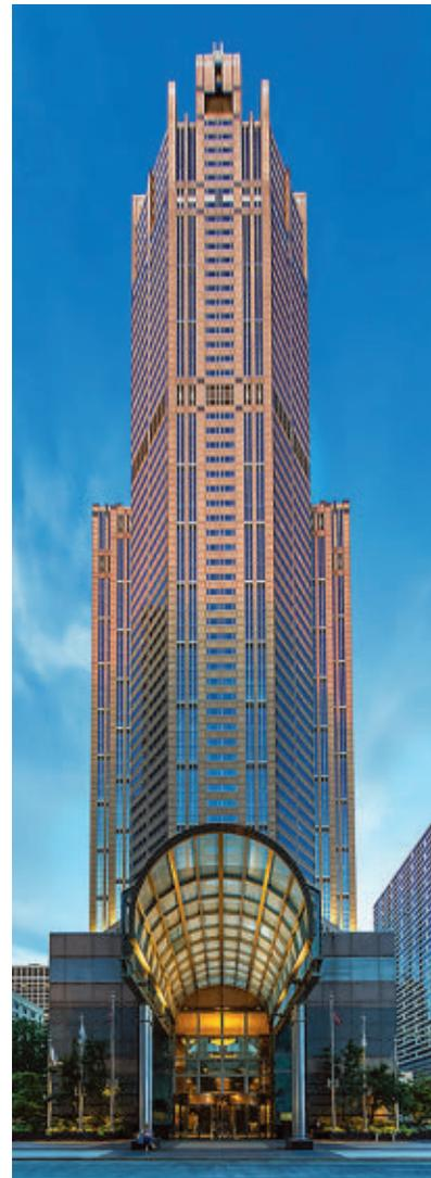
Zeller Realty Group's upgrade of the HVAC controls at 311 South Wacker Drive in Chicago's West Loop submarket has reduced HVAC energy use by 30 percent while improving tenant comfort. The 65-story, 1.4 million-square-foot tower has been dubbed "the smartest energy retrofit in Chicago."
